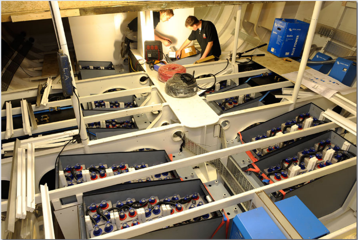
Photo 1: Victron equipment is being installed at the bottom of the yacht.
